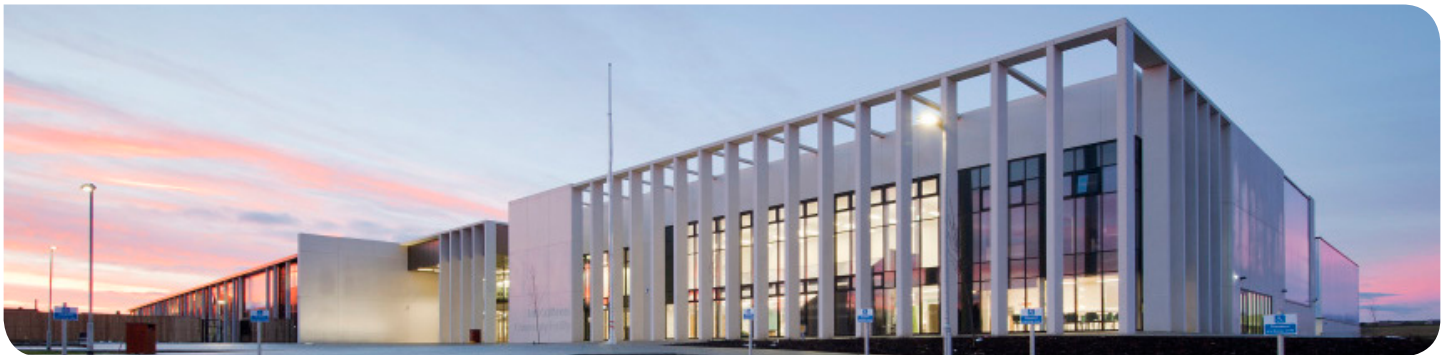
Photo courtesy of Donald MacLaren, Morrison Construction.
