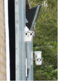
Vicom carried out a detailed site survey and capability test to ensure that the site could be monitored both day and night. Due to the dual lens capabilities and hemispheric models, the entire site was designed to be secured using just 6 cameras. The system is also integrated alongside IP Access Control, Intruder Alarm and Public Address Systems which are remotely monitored 365 days a year by an NSI Gold Alarm Receiving Centre (ARC).
