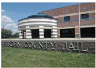
Bergen County Jail 820 MOBOTIX Cameras, U.S.A.
