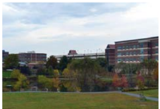
Valley Health Hospital 100+ MOBOTIX Cameras, U.S.A.
