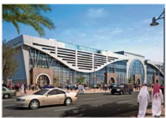
Barwa Commercial Avenue 1,840 MOBOTIX Cameras, Qatar
