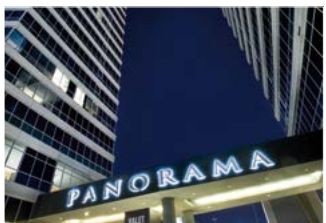
Panorama Towers 137 MOBOTIX Cameras, U.S.A.
